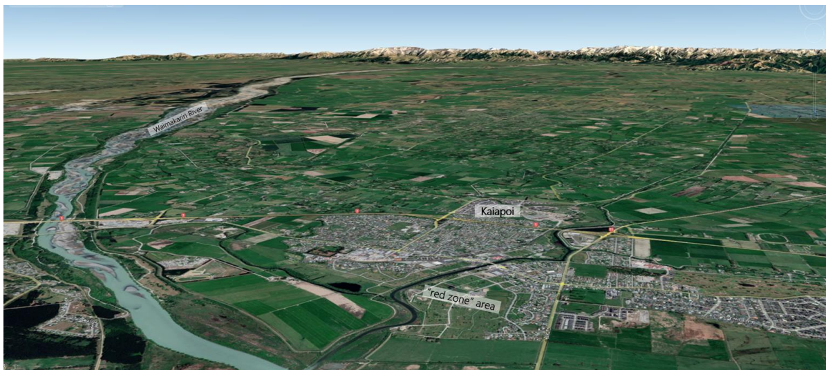
Figure 2: The area around Kaiapoi has extremely low topographic relief making it susceptible to widespread flooding. Areas of the town are part of a "red-zone" which have been retreated from due to liquefaction during the 2010-11 Canterbury earthquakes, which increased flood risk.
