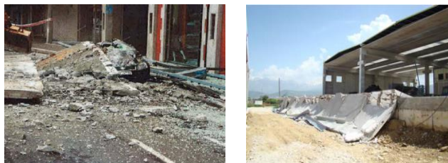
Fig. 9 – Damaged panels [2,10]
