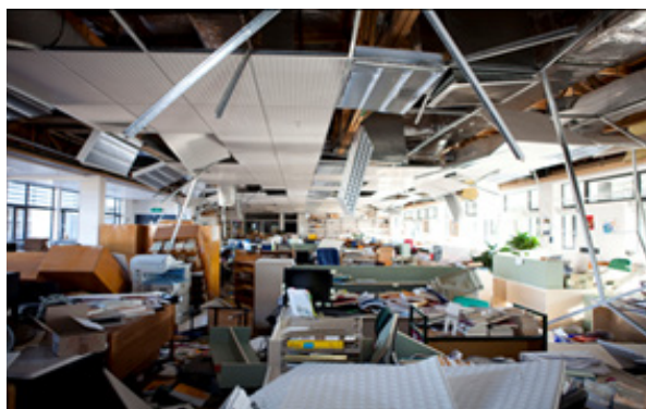
Figure 1: Illustrating damage to non-structural elements observed in the Canterbury earthquakes (from Dhakal, 2010)
